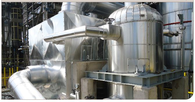
Thai refining and petrochemicals company IRPC replaced a shell-and-tube reboiler with an Alfa Laval Compabloc in order to use waste heat as heat source for a sulfolane stripper column instead of steam. This resulted in an annual reduction of 1,300,000 Euro in steam costs.
