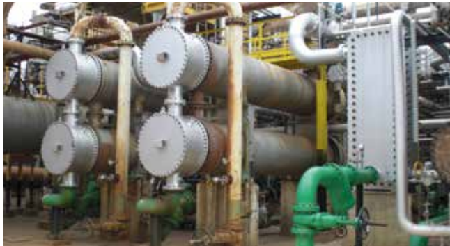
With its compact design, compared to a shell-and-tube heat exchanger, Compabloc can be installed where floor space is limited.
